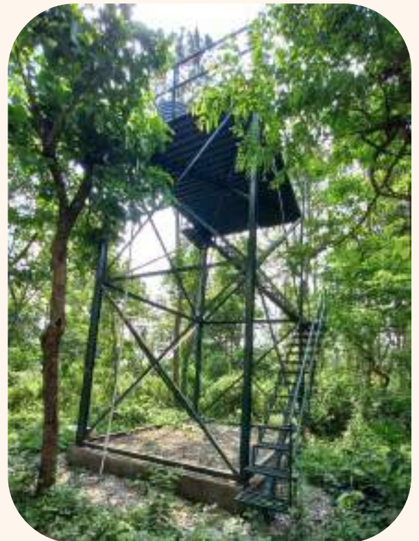
Fig: Construction of Central tower for water tank and water line
