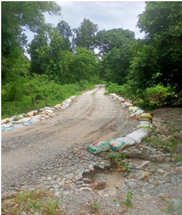
Use of gunny bags and RBM for road repair
