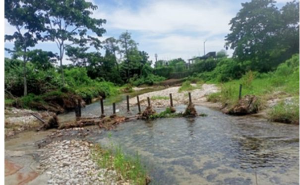
MS joists constructed across river
