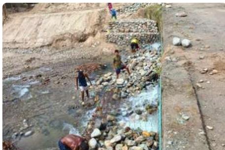
De-siltation of Jhora (Part-I) at NBWAP
