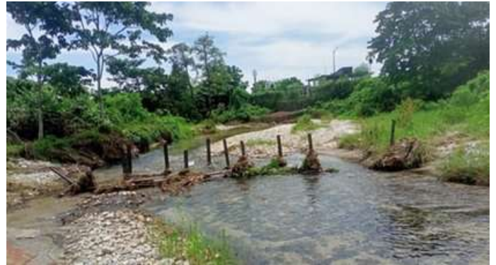
MS joists constructed across river
