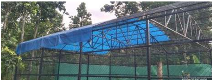
Tarpaulin cover at lion shelter
