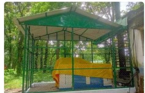
Extension of Generator Room at NBWAP
