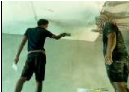
Maintenance: Painting of Tiger night shelter
