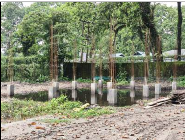
Initiation of two storied staff quarters
