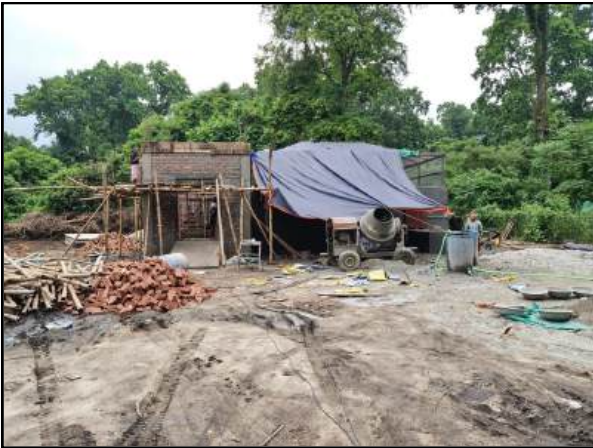
Initiation of animal rescue/quarantine center (night shelters & kraal) construction
