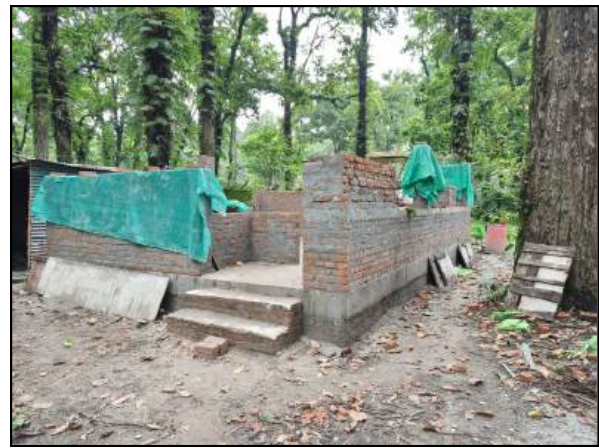
Initiation of security staff quarters
