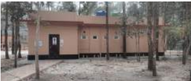
New Visitor's Toilet Block Inaugurated with Additional Amenities includes a changing room, wash basin, electric hand dryer, 15 additional latrines, and urinary chambers to provide a more comfortable experience.
