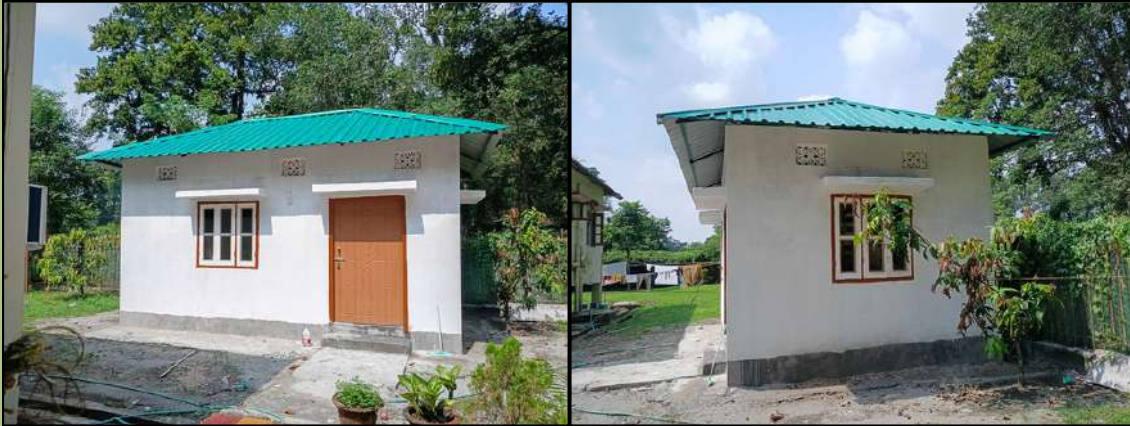
Construction of Guard room at BLD 1
