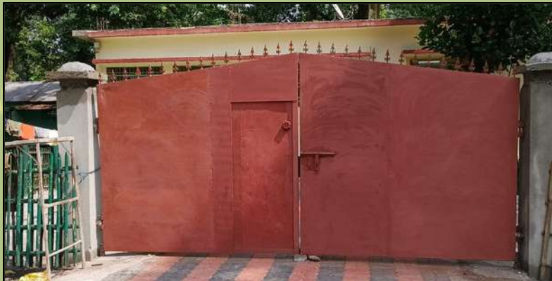
Compound gate repairing at R.O. quarter
