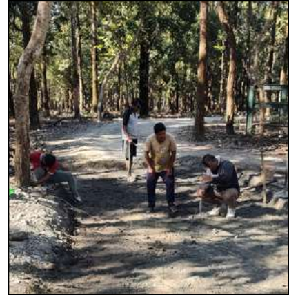
Repair and carpeting of the roads at safari area.
