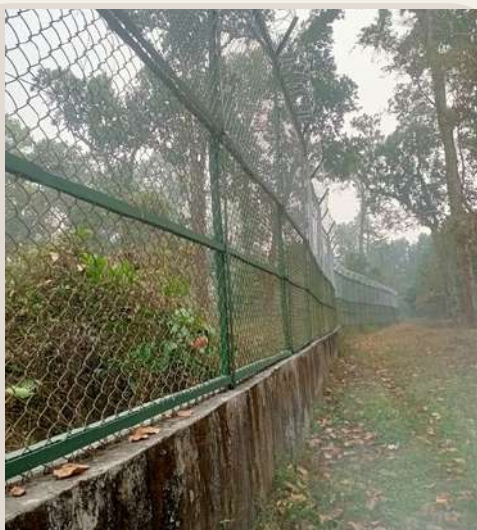
Vertical extension for existing herbivore fencing for conversion to carnivore boundary fencing (L-1300.00 m at NBWAP)
